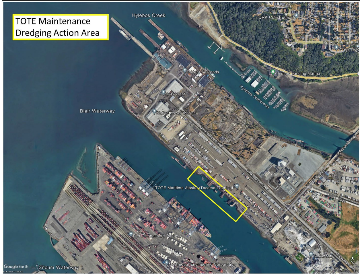
Figure 1. TOTE Maritime Alaska Terminal Action Area, Blair Waterway, Port of Tacoma (GoogleEarth).
