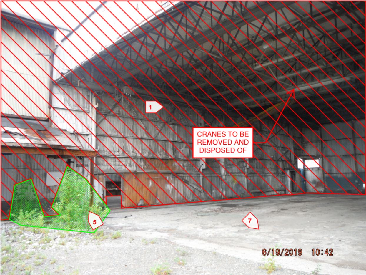
Figure 16 – 1110 Alexander Avenue Building Demolition Interior Photograph
