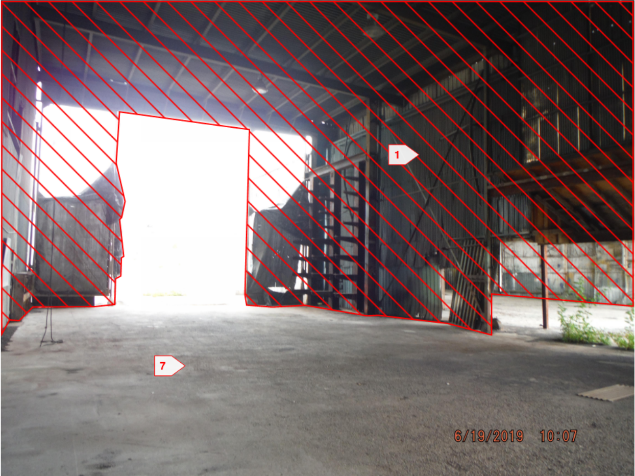
Figure 13 – 1110 Alexander Avenue Building Demolition Interior Photograph
