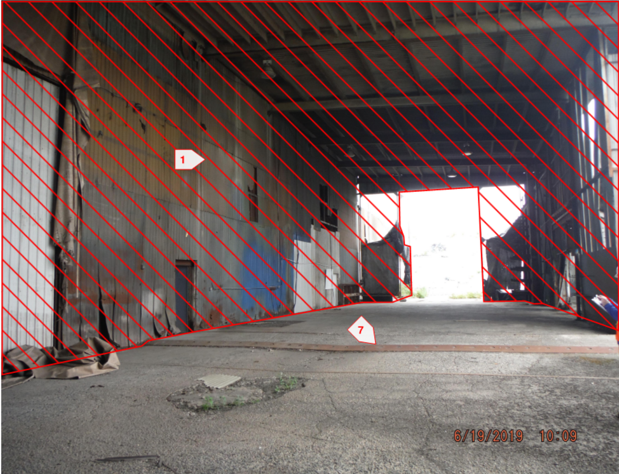
Figure 15 – 1110 Alexander Avenue Building Demolition Interior Photograph
