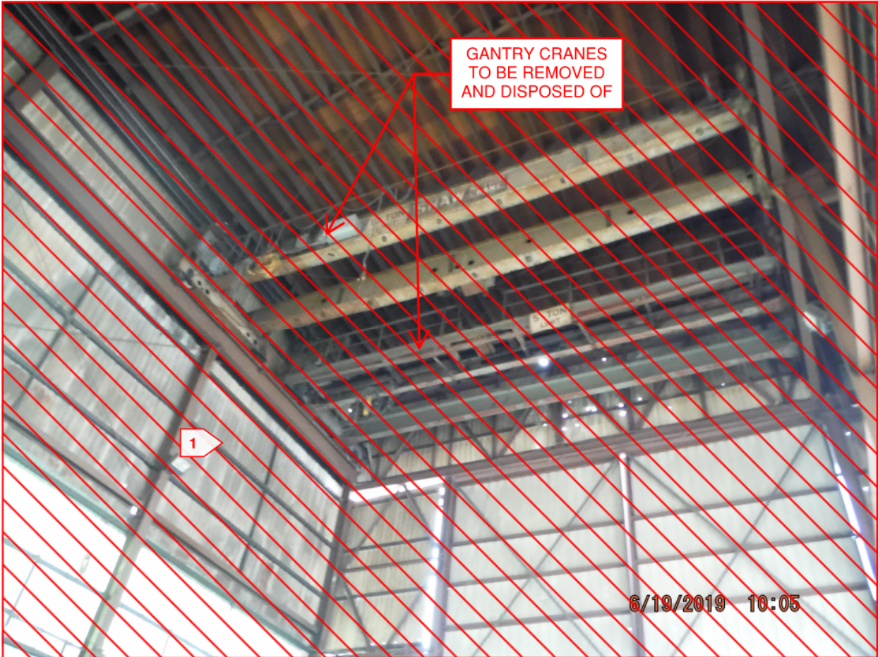
Figure 11 – 1110 Alexander Avenue Building Demolition Interior Photograph
