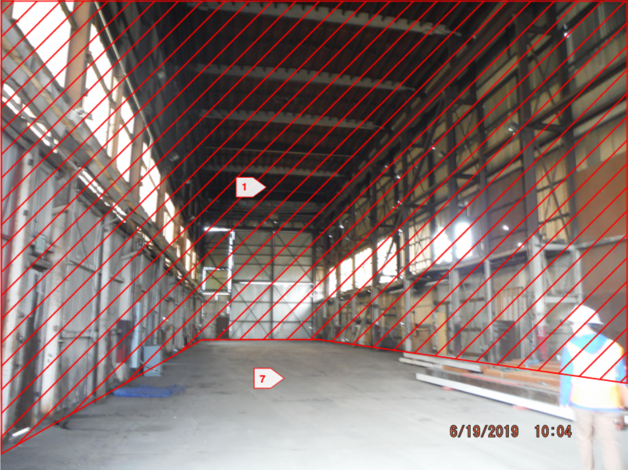
Figure 9 – 1110 Alexander Avenue Building Demolition Interior Photograph
