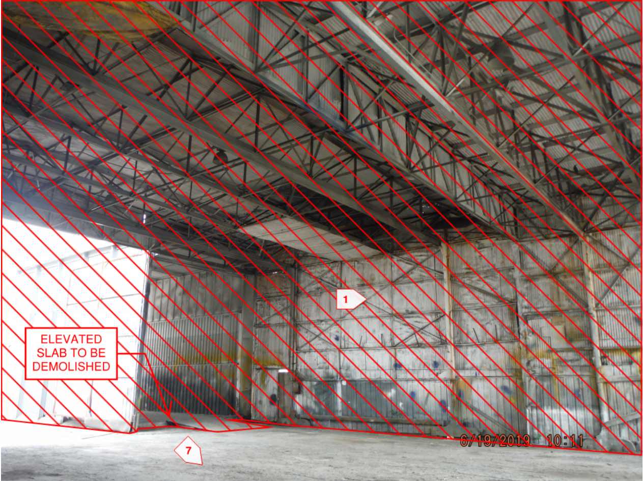
Figure 17 – 1110 Alexander Avenue Building Demolition Interior Photograph
